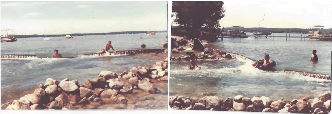
Figure 1.2.3. The outlet at Cut River, during a period when the full dam structure was not in place.
