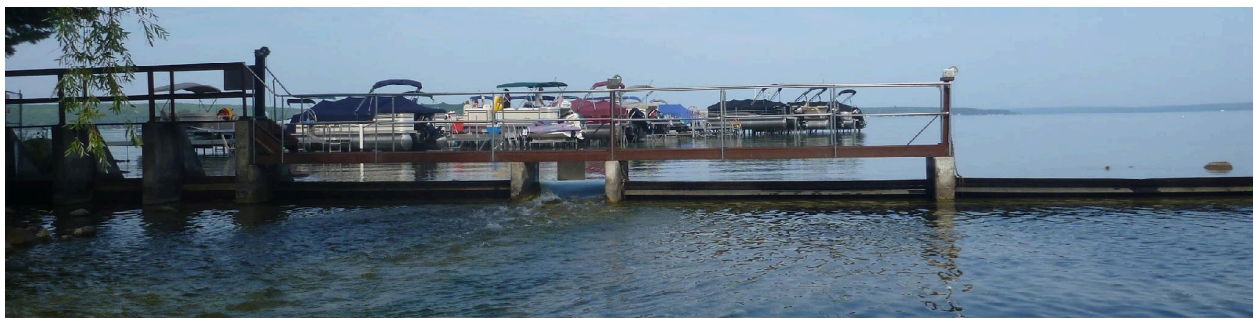
Figure 1.2.1. Image of the 2015 outlet control structure looking toward Higgins Lake from the Cut River. The low flow structure is in the center of the picture.
