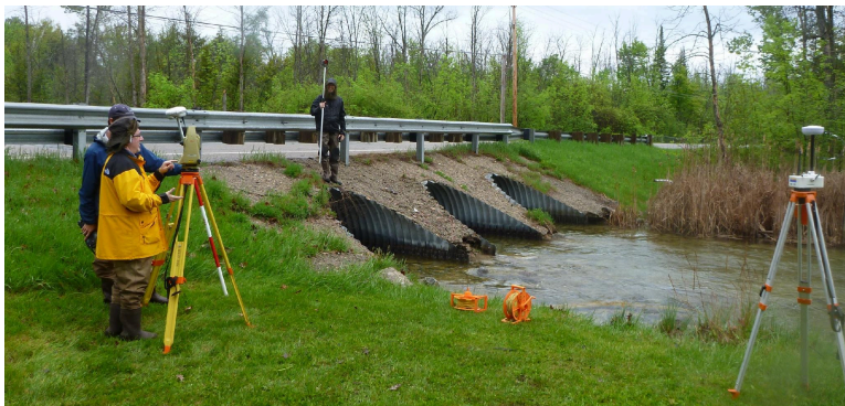
Figure 1.2.4. Photo of GPS and total station survey set up along the Cut River at the culverts under East Higgins Lake Road.
